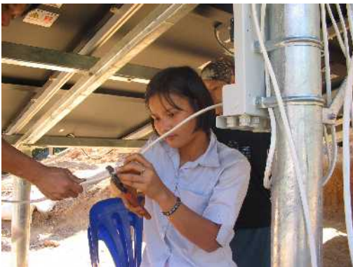
Naw Priscilla helps wire the combiner box together
