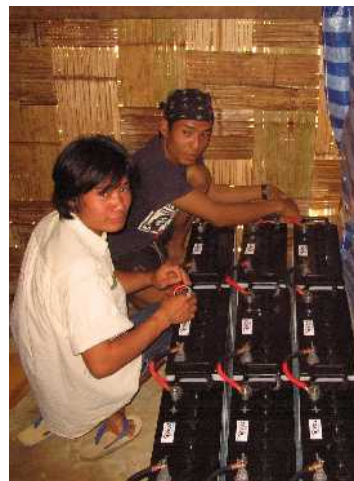
Saw T'Nar Tu Saw and Saw Sundry wire the batteries together
