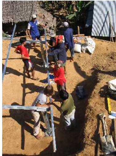
The team begins to assemble the PV structure
