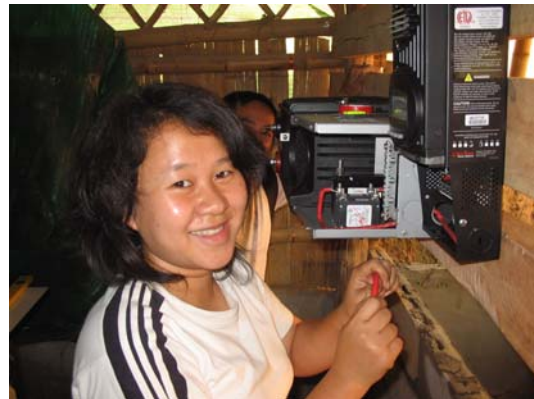
Naw Si Si Poe, ESP teacher, wires the inverter and charge controller.
